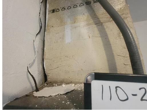
110-2 Duct Mastic Typical Interior HVAC
